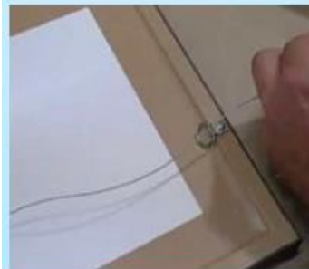
Secure quality TAPE to seal the gap between frame & back
